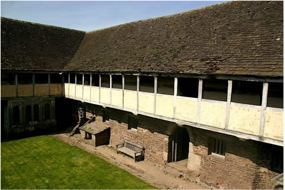
Windows overlooking the courtyard
