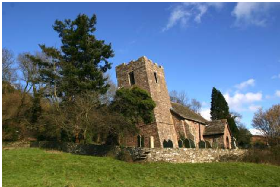
The leaning tower of Cwmyoy Church
